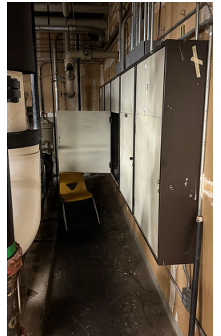
Existing Controls: Siemens APOGEE Automation Digital/Analog Input/Output
