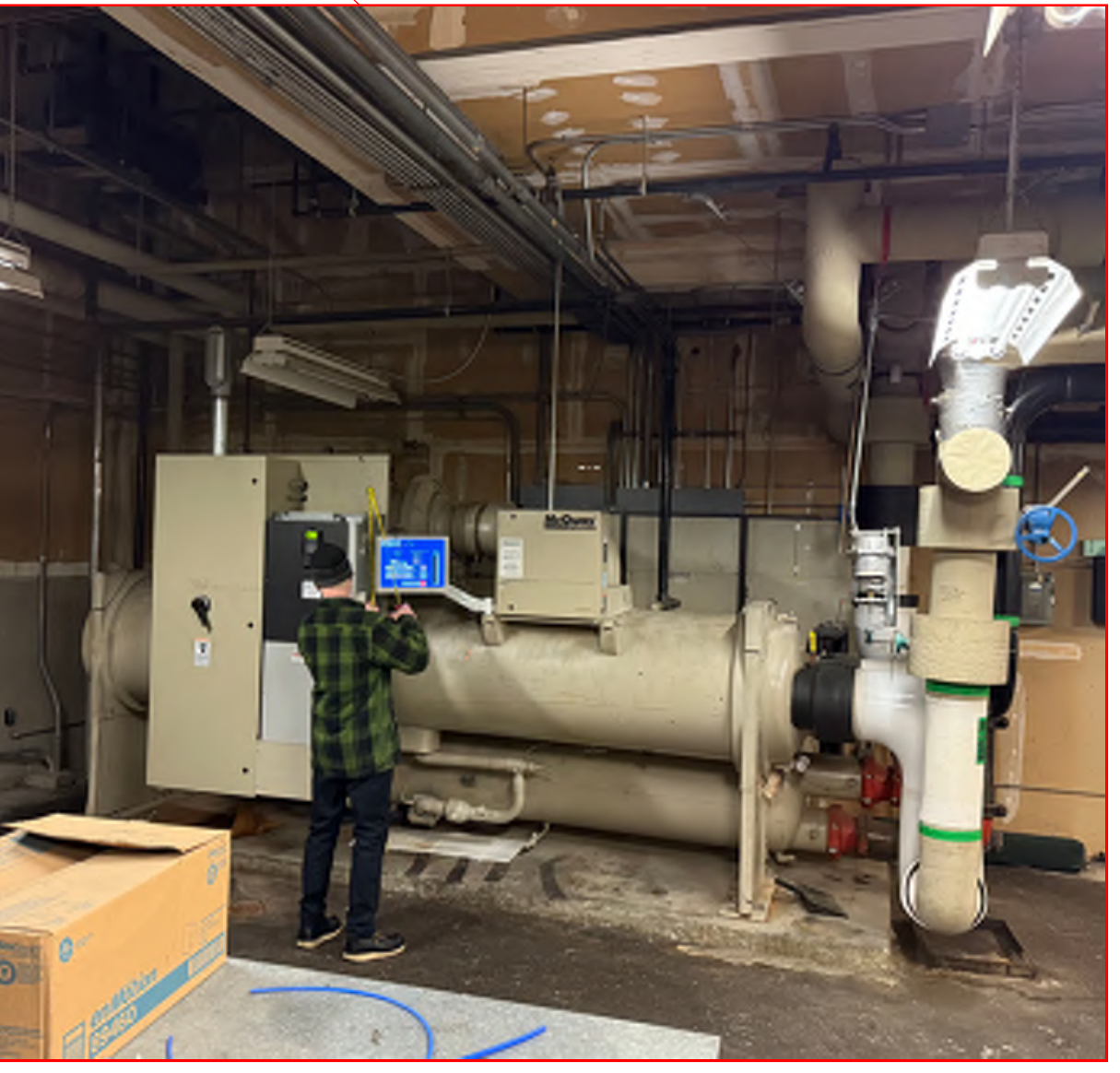
Existing Chiller: 300-ton McQuay WSC063S37 centrifugal. Concrete Pad: 4'-9" W x 14'-6" L x 4" H
