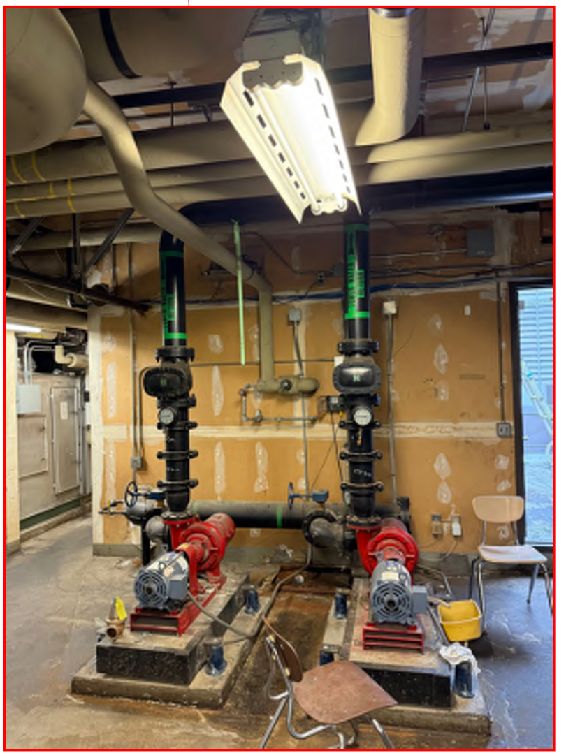
Existing Tower Pumps: Armstrong Model 65-7609, 10 HP motors @ 230/460 3ph
