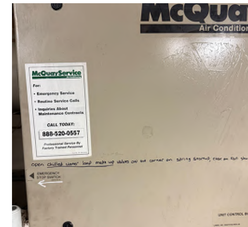
CHILLER DISCONNECT AND EMERGENCY STOP SWITCH
