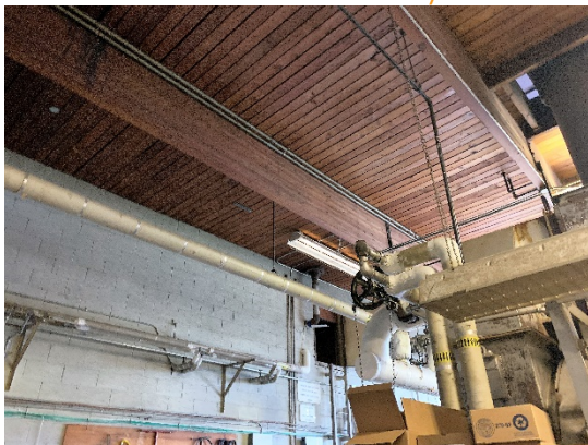
Figure 18: Boiler Room Roof with Glulam Beams and Straight Sheathing Roof
