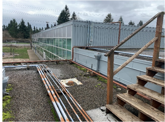
Figure 11: Roof Interface Between High and Low Roofs
