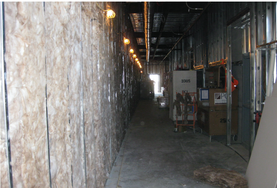
Above: Separation wall keeps students and construction from interacting throughout the process. Noise is minimized with temporary insulation. Above Right: Fencing and appropriate fence signage directs foot traffic and keeps the separation of construction site activities and students.
