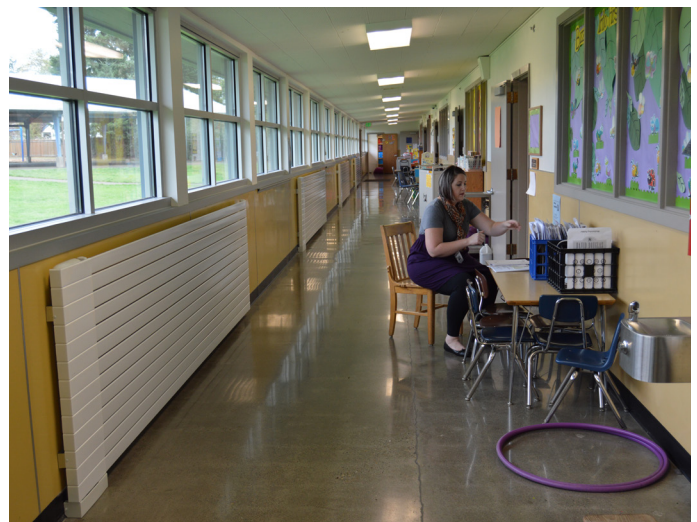
Polished concrete floors were an excellent choice for durability
