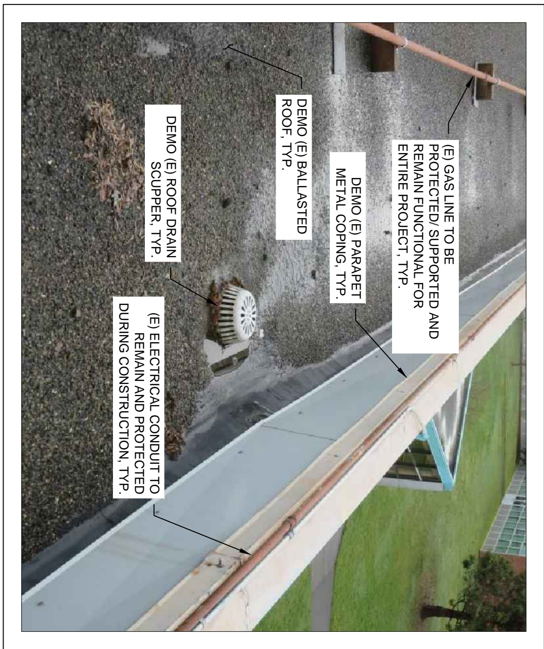
3 D1.1 ROOF DRAIN ELEVATION NTS
