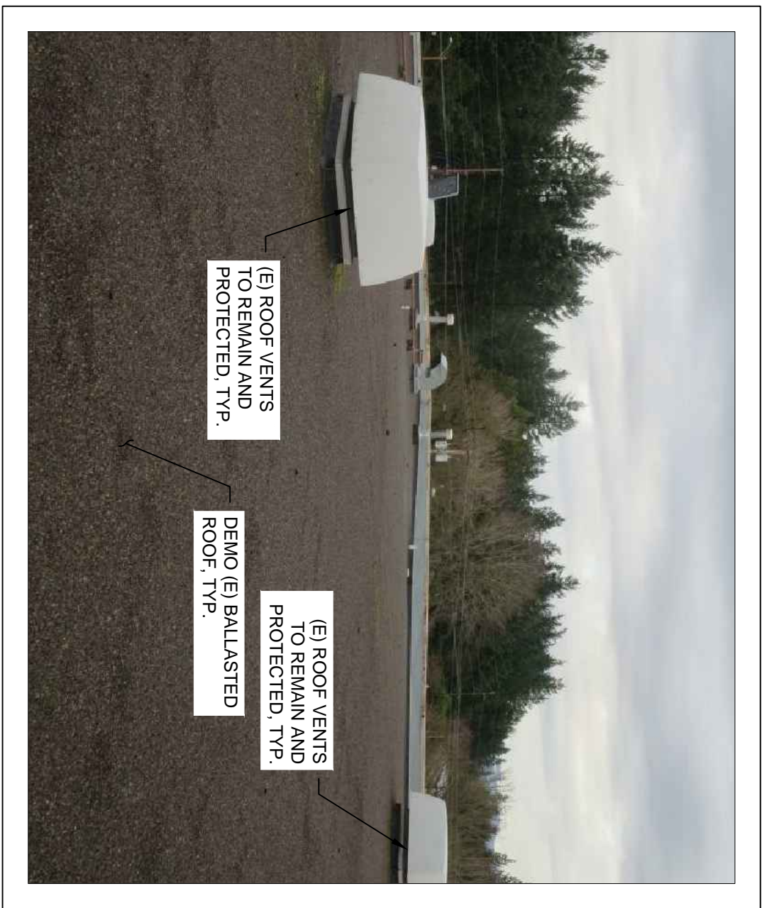
5 D1.1 ROOF VENT ELEVATION NTS
