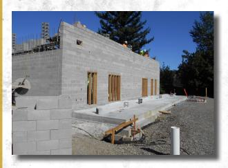
The gym walls have started going up! Our crew uses CMU (concrete masonry unit) bricks to build the walls of the gymnasium. The tall CMU walls paired with the strong roof trusses are what allows a gym to be an open structure. We wouldn't be able to play sports as easily if there were columns in the middle of the gym, would we?
