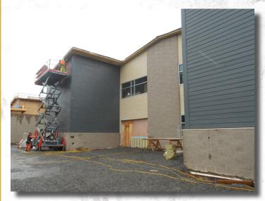
Windows and door frames are being installed throughout the building. On the exterior, the block and wood siding are continuing to go up, giving the new school its final look. Additional work on the interior includes running electrical wires, insulating ductwork, and installing insulation and sheetrock in the classrooms of area 3.
