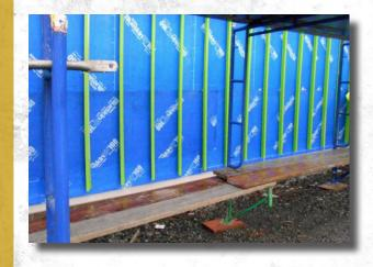
In order to keep the building dry and warm, a couple of important layers have to be installed before the outside brick can go on. The blue in the picture to the left is the weather barrier that keeps the building dry. The green strands you see, called girts, is where the insulation will go to keep the building warm. Our crews will then add the brick to the outside, which will give your new school it's finished exterior look.
