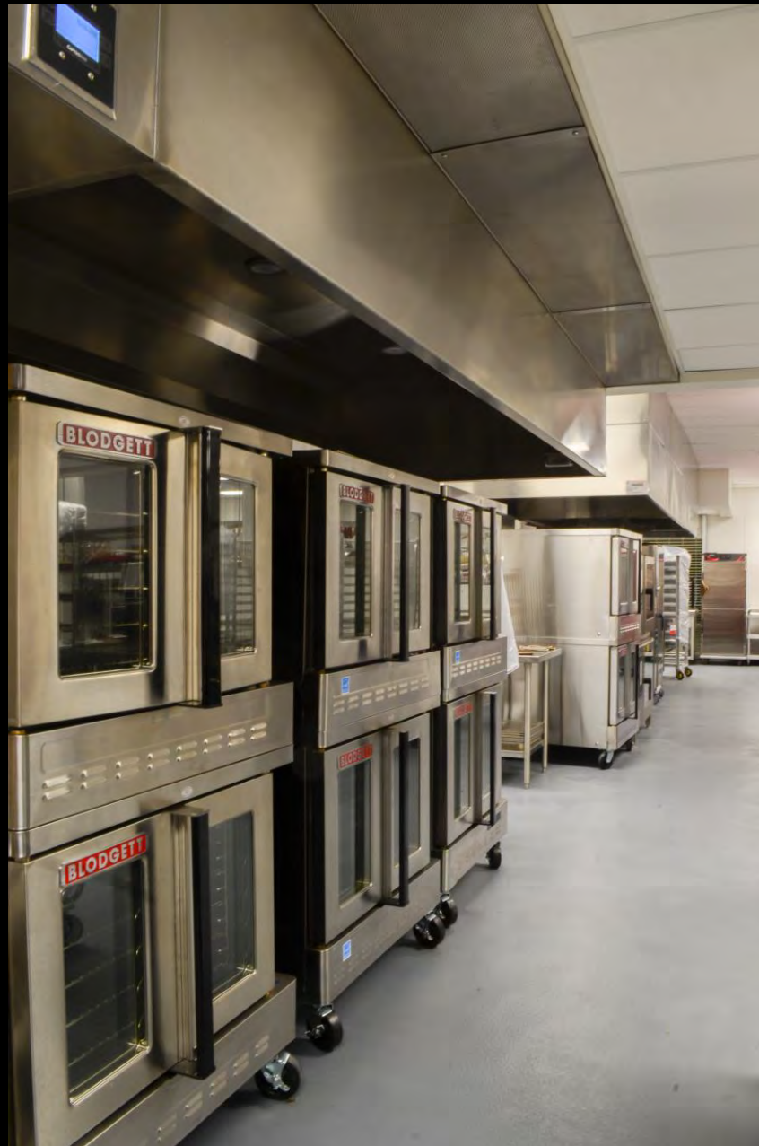
Reynolds High School – March 2019 – Kitchen
