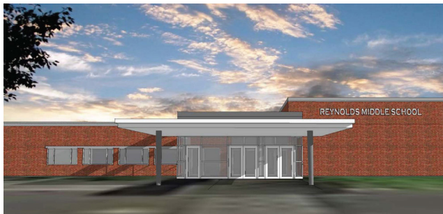
Reynolds Middle School Secure Vestibule Entrance
